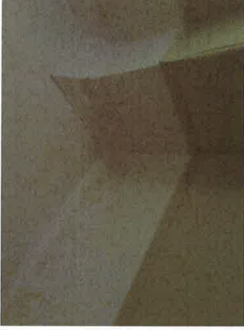
24. Front room cornice detail
