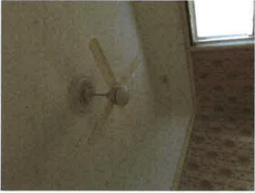
27. Bedroom ceiling detail
